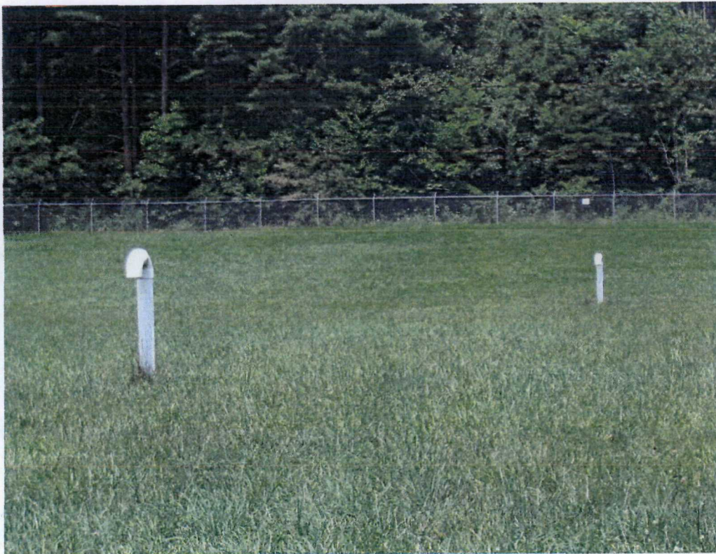
Photo #4 - Acid Pit Vent System
