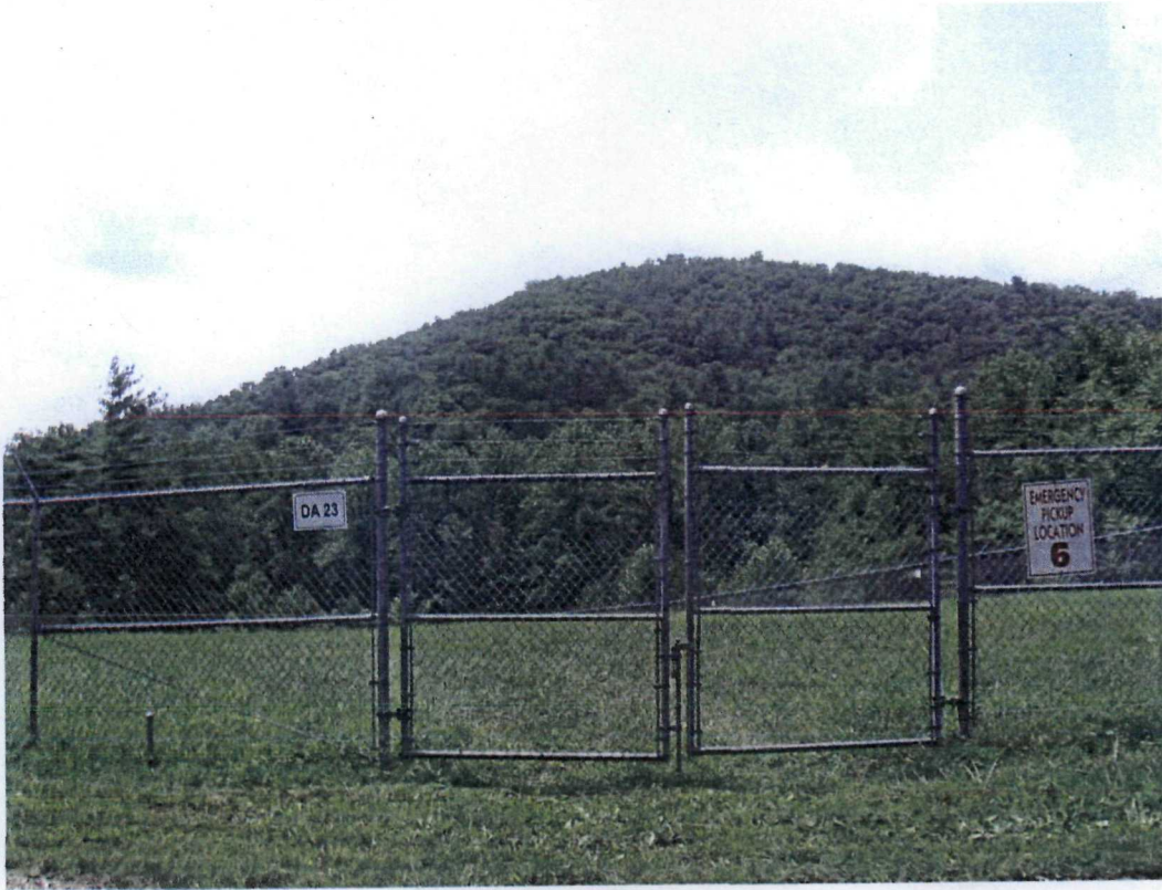
Photo # 1 - DA-23 Fence and Cap
