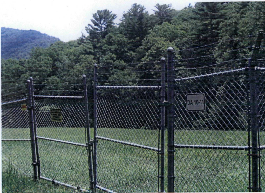
Photo #2 - DA 10/11 Fence and Cap
