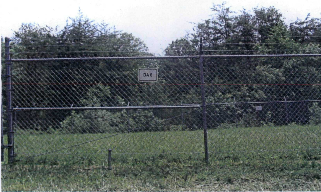
Photo #5 – DA 6 Fence and Cap
